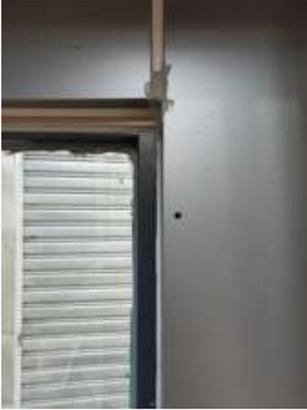
Figure 3: 8mm hole at 3/4 window height
