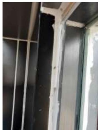
Figure 8: 8mm hole at 3/4 window height in caulking
