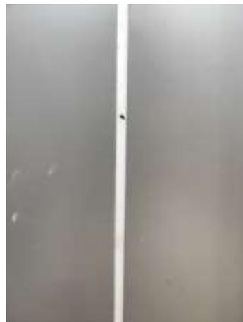
Figure 6: 8mm hole in panel joint caulking
