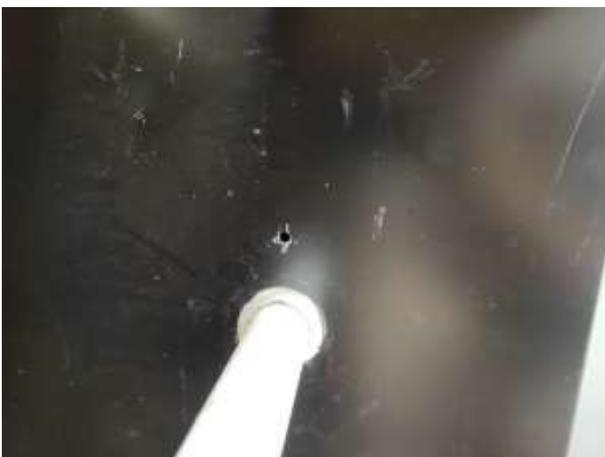
Figure 7: 8mm hole above pipe penetration
