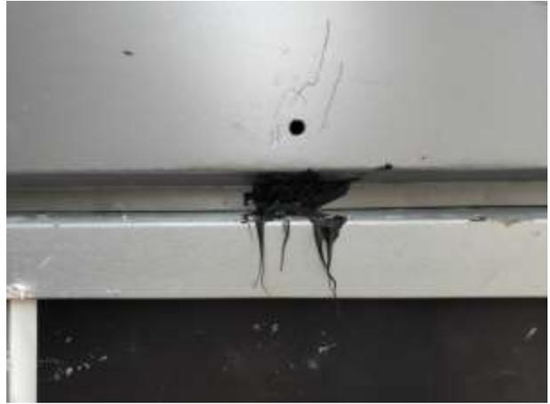
Figure 4: 8mm hole above horizontal control joint
