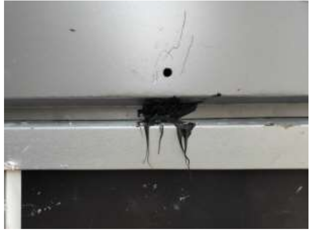
Figure 4: 8mm hole above horizontal control joint
