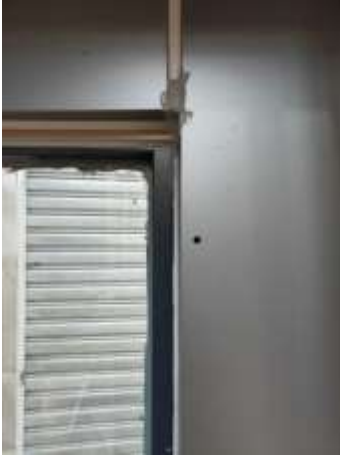
Figure 3: 8mm hole at 3/4 window height
