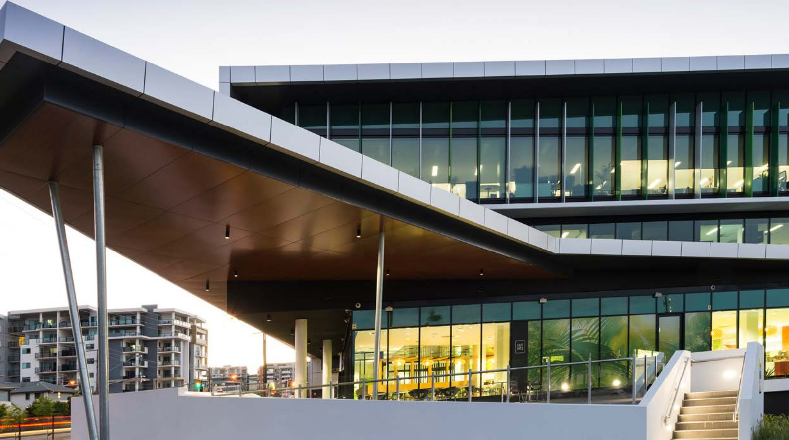
CHERMSIDE NORTHERN REGIONAL BUSINESS CENTRE & LIBRARY, QLD
