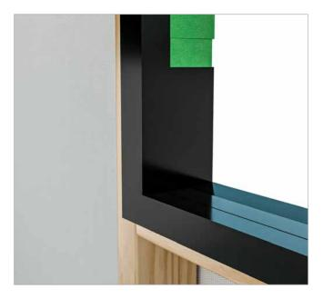
**5. APPLYING THE FAÇADE TAPE TO SILL** Repeat this process for the rear edge of the frame, then do the right a left hand side and finish off with the header.
