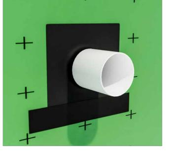
**4. SEALING COLLAR EDGE SEALING** Begin by applying the sarking tape along the bottom edge of the collar. Ensure that it forms a good bond onto both the collar and the membrane.
